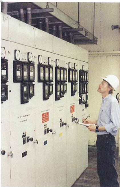
3. Manual megger readings have been replaced by in-line testers that automatically monitor the condition of winding insulation in critical motors (above)
